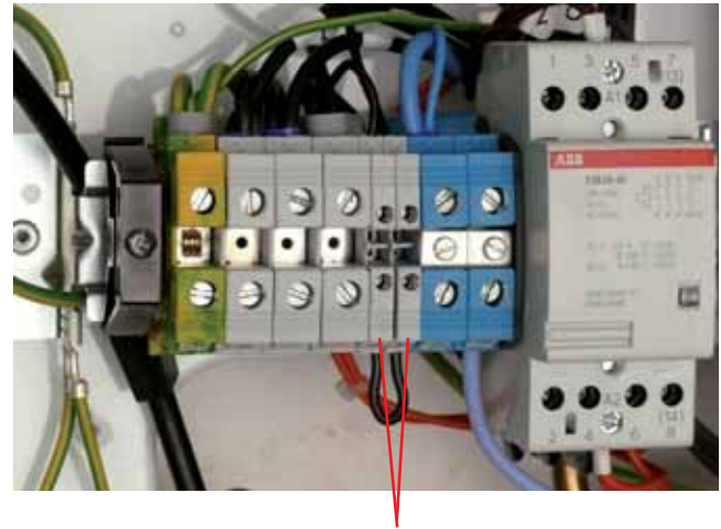
Terminals for connecting an emergency thermostat for floor heating (009642)
